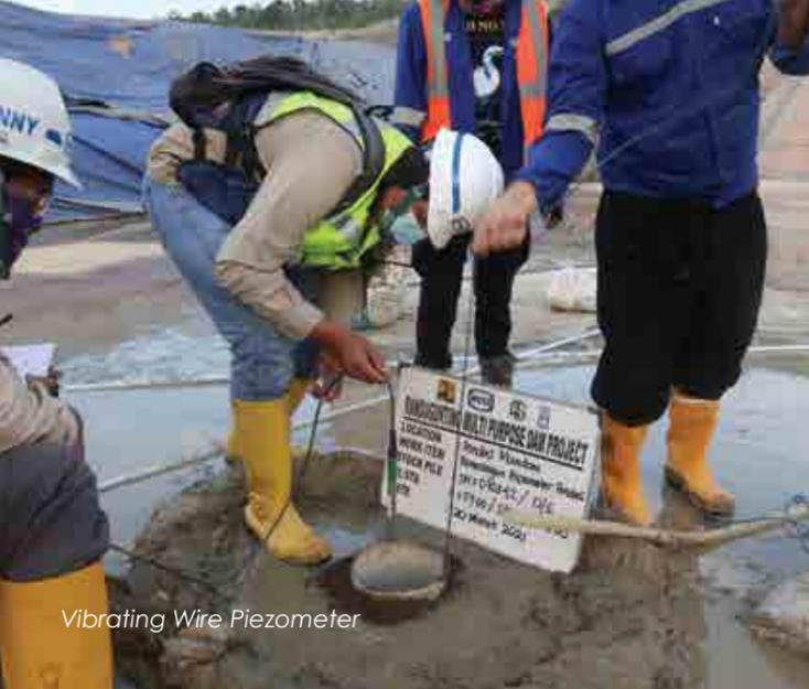
Vibrating Wire Piezometer
